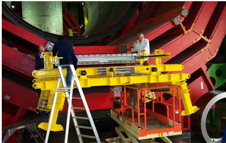
Fig. 16. Installation of a MB1 chamber with final tooling
