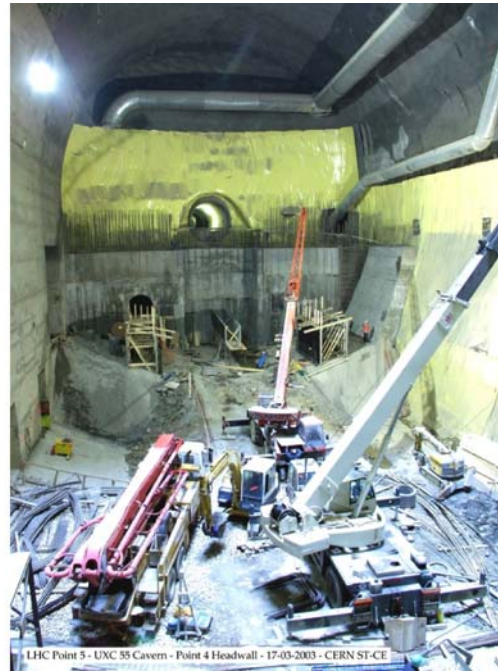
Fig. 2. Concreting work in the two underground caverns: USC55 ( service cavern on the left ) and UXC55 ( Concreting work in the two underground caverns: USC55 (service cavern on the left) and UXC55 (experimental cavern on the right) )
