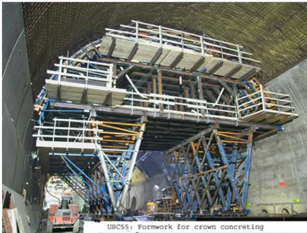
Fig. 2. Concreting work in the two underground caverns: USC55 ( service cavern on the left ) and UXC55 ( Concreting work in the two underground caverns: USC55 (service cavern on the left) and UXC55 (experimental cavern on the right) )
